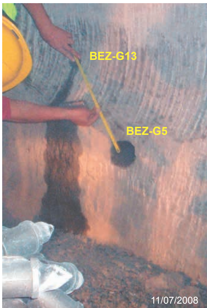
Fig. 6-19: Views of the Ga08 front at GM 159: the end of BEZ-G13 was opened July 11 when the upper part of the gallery was excavated (left photo, 11/07/2008 evening), the end of BEZ-G12 was opened July 12 when the lower part of the gallery was excavated (right photo, 14/07/2008 evening).
