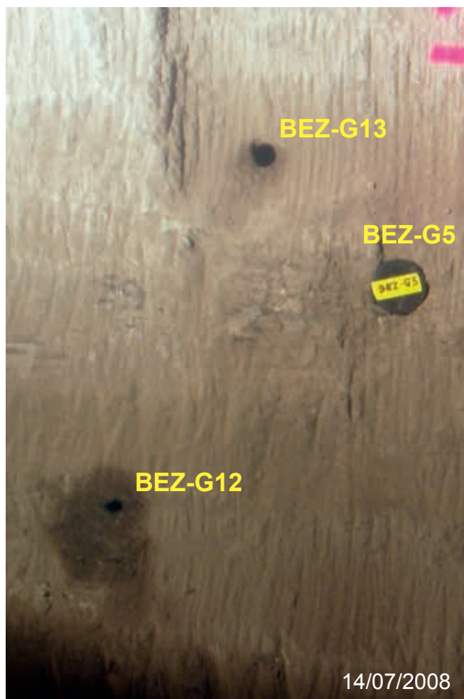
Fig. 6-19: Views of the Ga08 front at GM 159: the end of BEZ-G13 was opened July 11 when the upper part of the gallery was excavated (left photo, 11/07/2008 evening), the end of BEZ-G12 was opened July 12 when the lower part of the gallery was excavated (right photo, 14/07/2008 evening).
