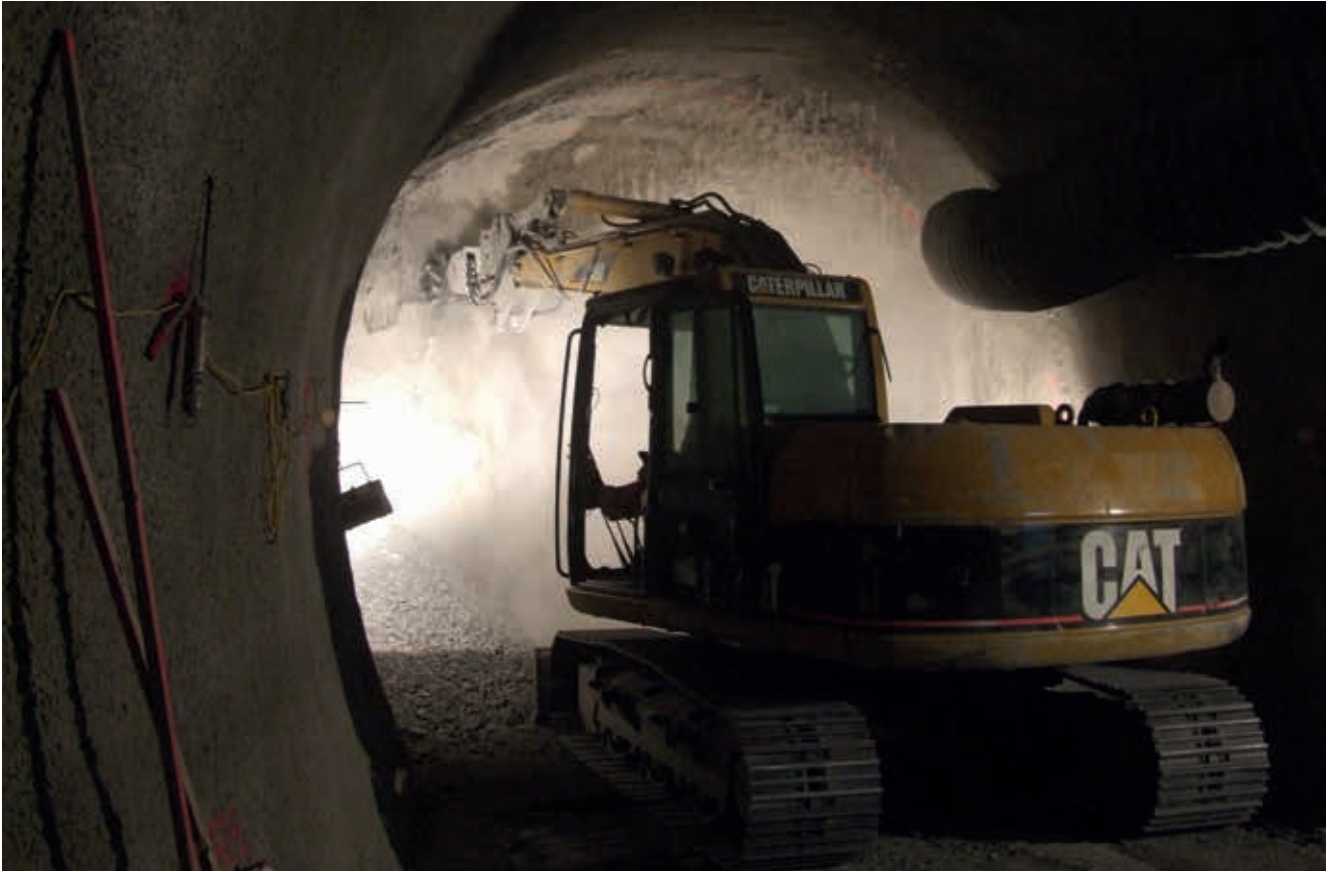
Fig. 2-2: A special type of excavation machine, i.e. a road header (hydraulic drum cutter Erkat ER 600) mounted on an excavator machine was used for the excavation.
